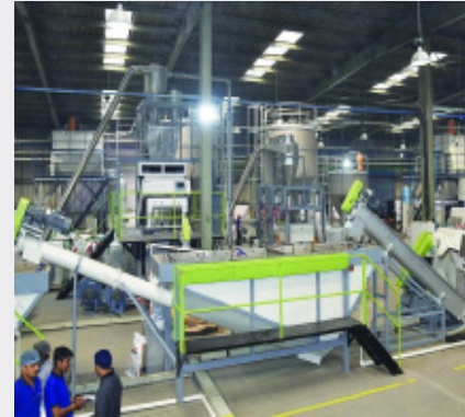
UFlex Recycling Plant, Noida (Inside View)
