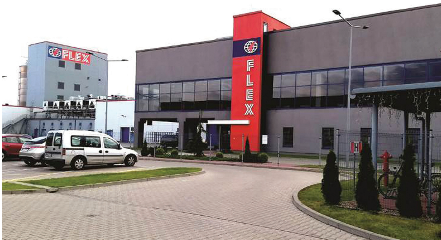
Uflex's plant in Poland
